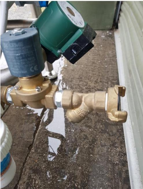
Permanent water fitting with automatic valve.
